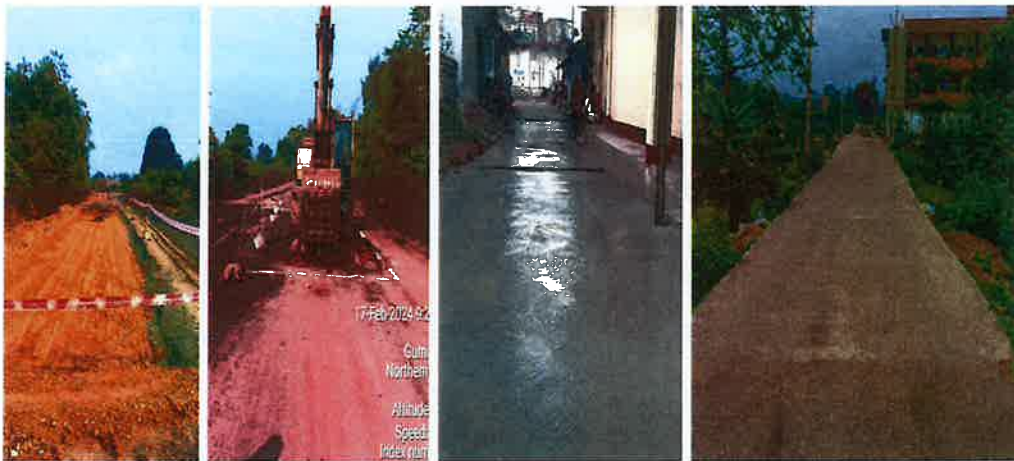
Ongoing Construction of Road at Derba
