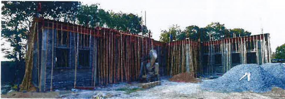
Ongoing Construction of Thelkoloji High School, Thelkoloji
