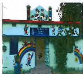
Anganwadi Center, Jhakarpada
